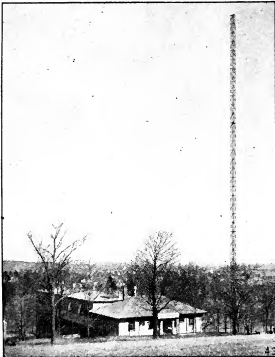
THE FIRST TOWER AT WGI
